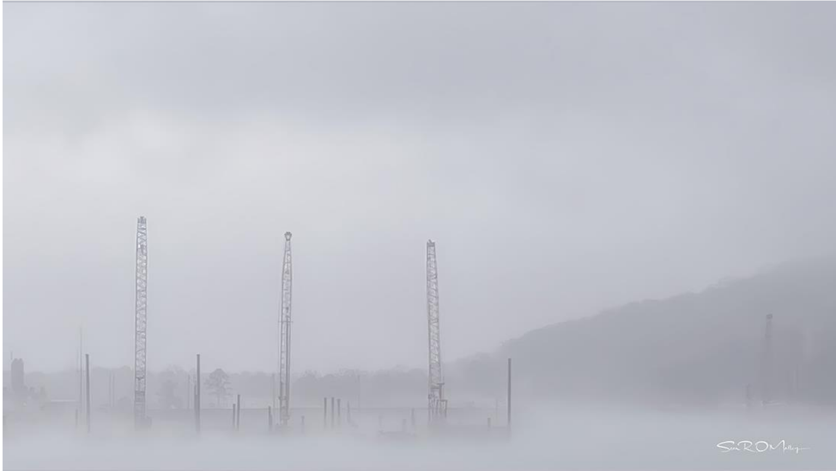
Sean O'Malley Ooltewah, TN 9 x 16 That Dam Project in the Mist $250
